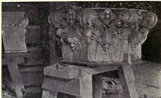
FIG. 59—CONCRETE CAPITAL FROM SAND MOLD, PARTIALLY CUT BY STONE CARVER
